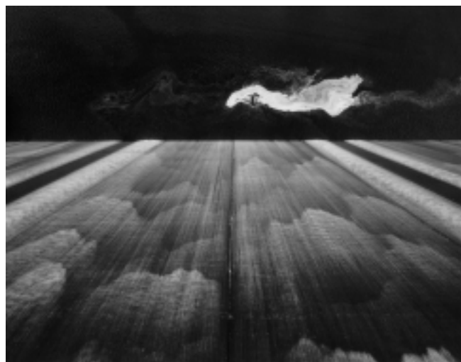
Grand coulee Dam, Douglas County, WA 1996
